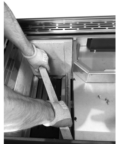
Fig. 68 - Remove the refractory material
