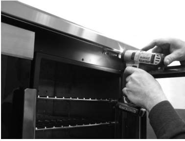
Fig. 71 - Screw removal
